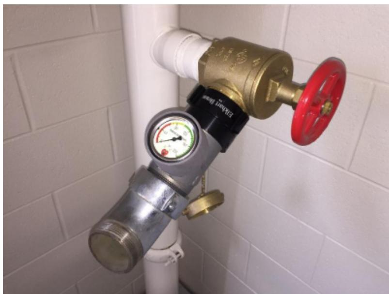
The above picture shows the hook up order on the standpipe. The inline pressure gauge goes on first. The ideal pressure we are looking for at the standpipe is 65psi. It will still work quite well at lower psi's, which is a reason we moved to 2 1/2" hose with a smoothbore.
