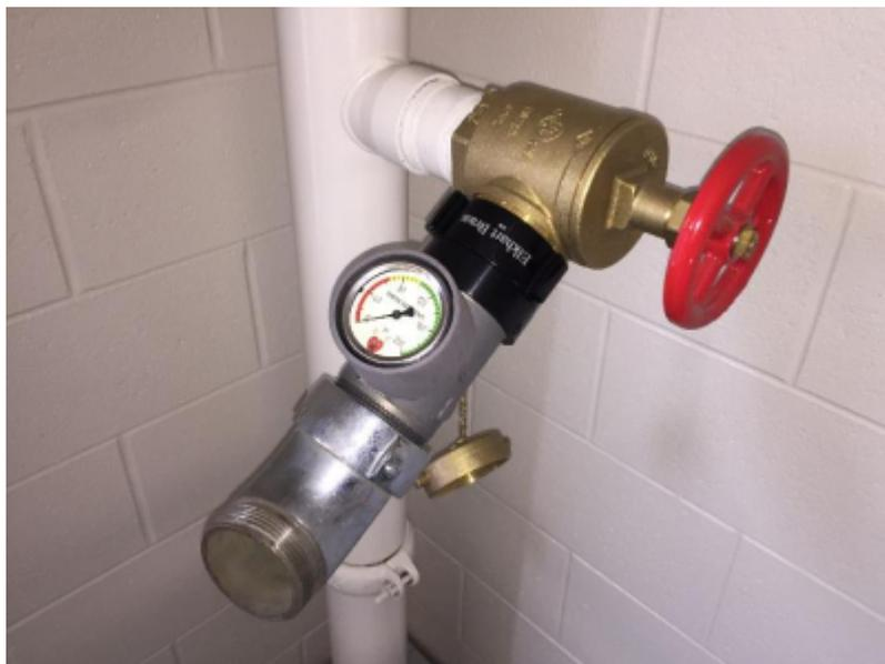
The above picture shows the hook up order on the standpipe. The inline pressure gauge goes on first. The ideal pressure we are looking for at the standpipe is 65psi. It will still work quite well at lower psi's, which is a reason we moved to 2 ½" hose with a smoothbore.
